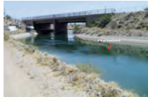
The CAP canal between Shea Blvd Bridge and Va Linda Bridge has subsided differentially by 2 ft. (Photo taken in 2001). Differential subsidence can cause flow reversal, damages to the channel lining and water leaks.
