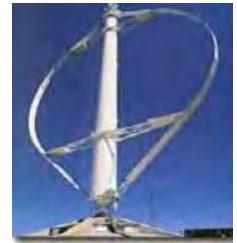
Fig. 1 The Classical Darrieus Wind Turbine installed by Hydro Quebec, CANADA
