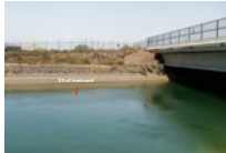
The CAP canal between Shea Blvd Bridge and Va Linda Bridge has subsided differentially by 2 ft. (Photo taken in 2001). Differential subsidence can cause flow reversal, damages to the channel lining and water leaks.
