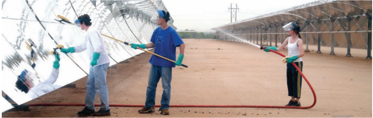
Engineering students “contact wash” large parabolic mirrors at the Arizona Public Service all-solar electric generating station in Red Rock, Ariz.
